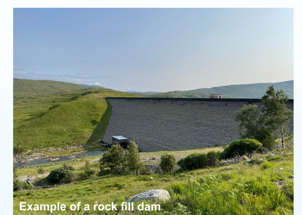
Example of a rock fill dam
