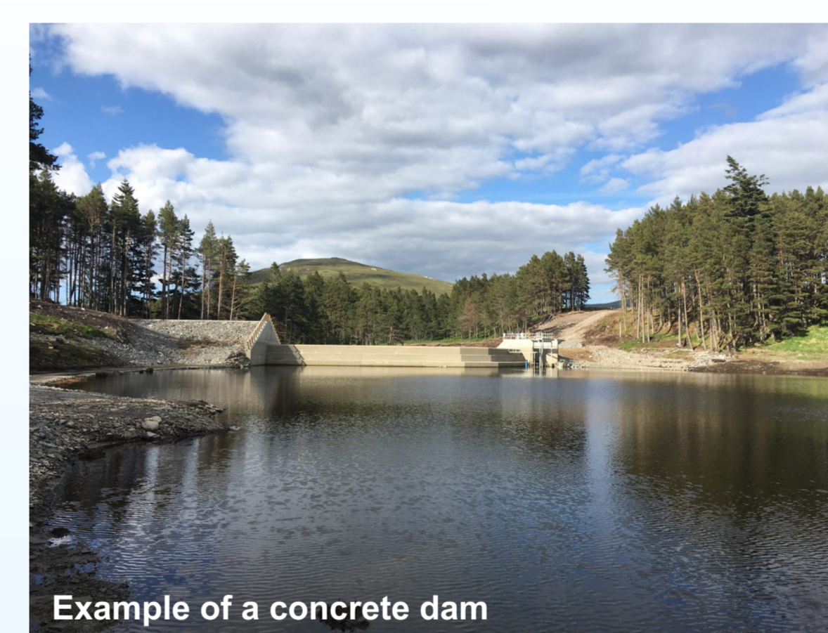
Example of a concrete dam
