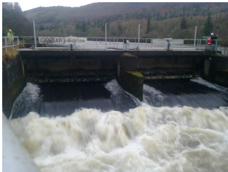
Image 1: SSE Renewables Outlet Sluice Structure on the East Bank at Ballindarroch (taken from Aecom 2016)
