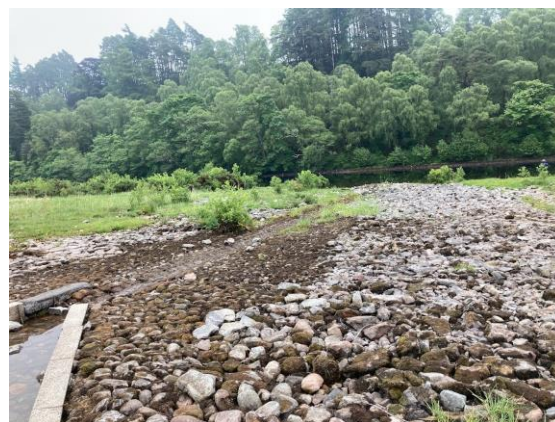
Plate 2: Smolt Pass (chute) flowing towards the River Ness with minimal flow and water depth across the waste weir during low loch levels.
