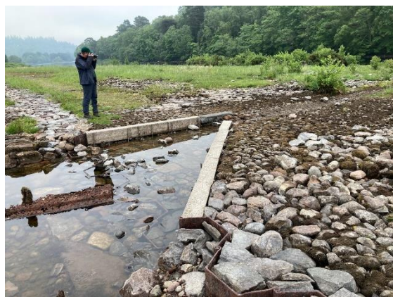
Plate 1: Smolt Pass (chute) entrance from the Caledonian Canal during low loch levels. Limited attraction for smolts to enter the bypass. Loch Level was 1.26 m on Foyers Gauge, well below typical mean low level 1.39 m). The chute had limited attraction for downstream migrating smolts with very little flow and water depth
