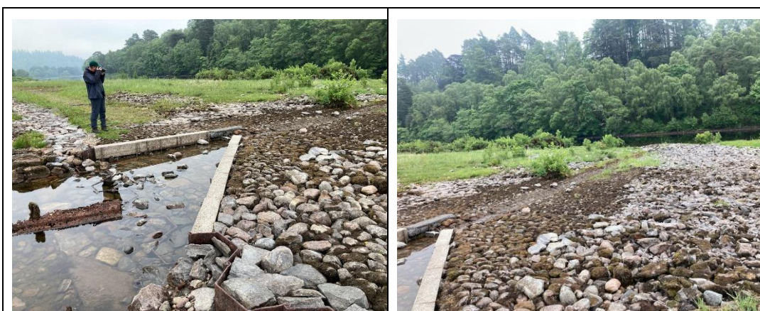
Plate 13.1: Smolt chute entrance from the Caledonian Canal. Limited attraction for smolts to enter the bypass.
