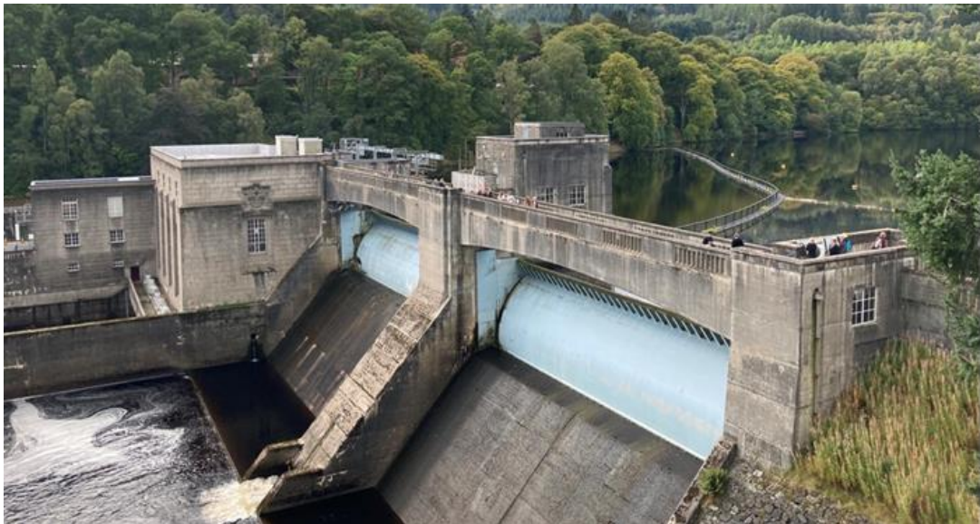
Plate 3.3: Example of a RCC Dam - Photo of Pitlochry Dam with Spillway (taken 2022)
