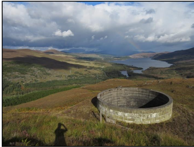
Plate 3.4: Example of a Surge Shaft
