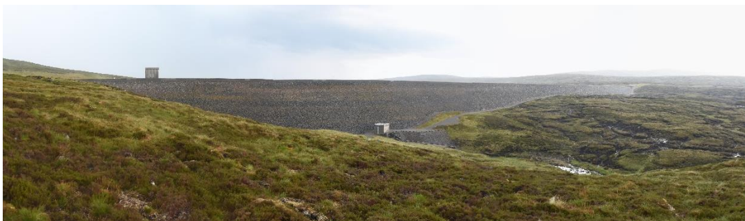
Example of a CFRD Dam - Photo of 'dryside' of Glendoe Dam (taken 2023)
