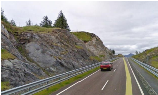
Rock Cuttings on the A830 near Arisaig
